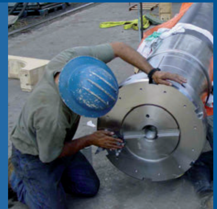
Delivering Becker spare parts
